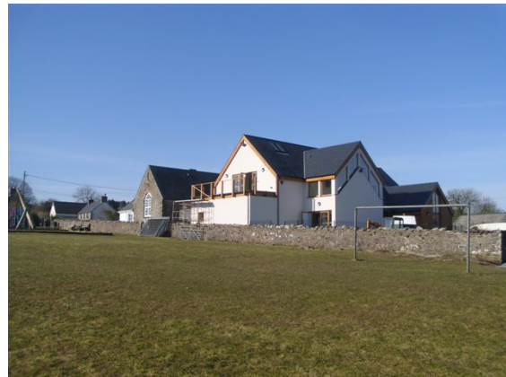
The renovated Canolfan Hermon
